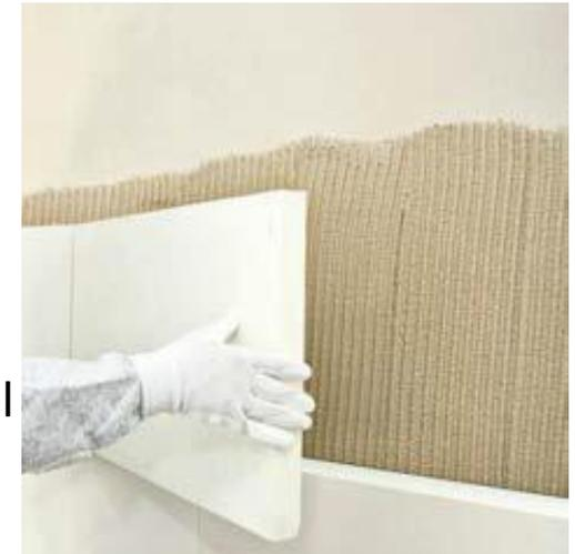
Pannello in aerogel e fibre
